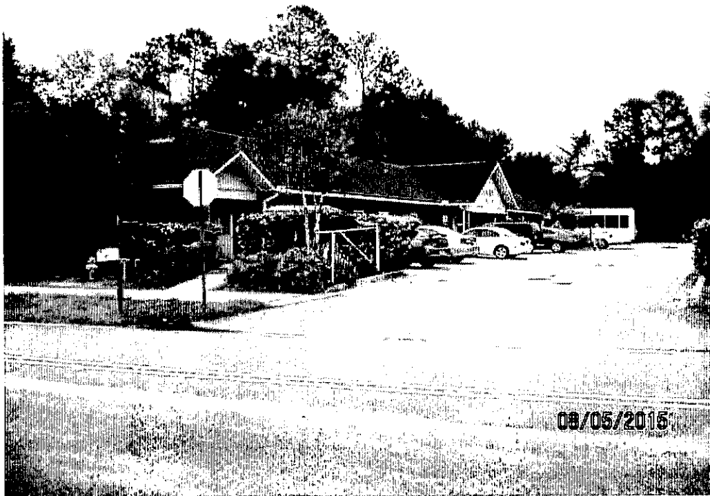
Existing commercial office across Cortez Road
